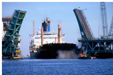
In 1996, the Julie N oil tanker spilled almost 180,000 gallons of fuel oil into the Fore River after striking the former Million Dollar Bridge while entering the harbor.
