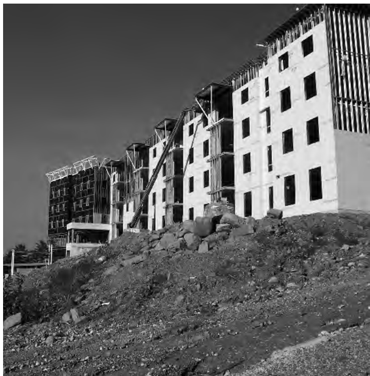
Work continues on the new dorm in Gorham.
