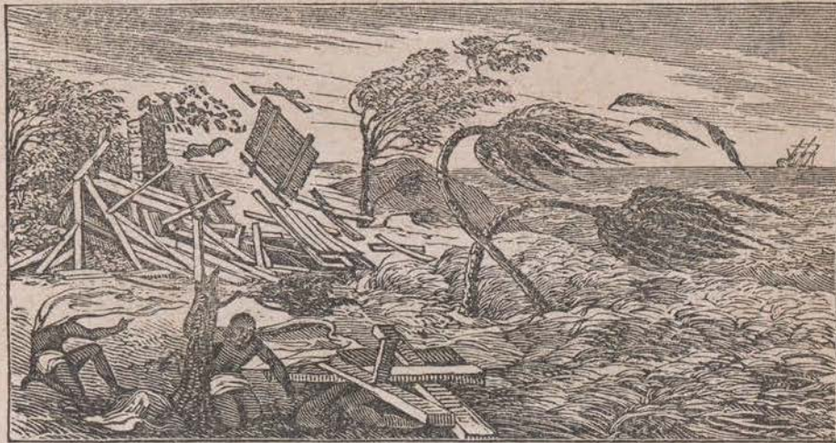
Hurricane in the West Indies.
