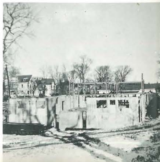
Lay The Foundation.
