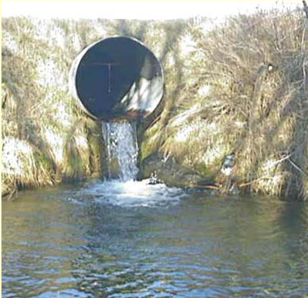
Scour downstream of undersized Culvert-ANR Photo
