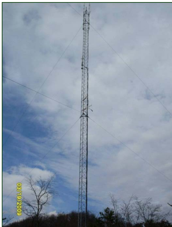
MET tower used for the Presque Isle project (picture courtesy of Solaya)
