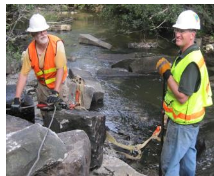
Workers attaching grip hoists to granite blocks in the Royal River
