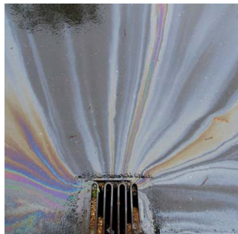
Impervious surfaces like roads and driveways channel pollutants into stormwater systems that discharge into the rivers and streams. Above, oil enters a storm drain.
