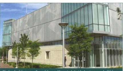
The facade of the top two floors of the map library is clad with aluminum panels. Of these panels, 104 have been etched with a projection of the world known as the Dymaxion Map. It was created in 1946 by the noted futurist and inventor Buckminster Fuller to represent the entire globe with minimal distortions. It may well be the largest such exterior map in the world.
