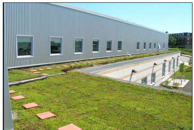
East End Community School Green Roof, Portland, Maine
