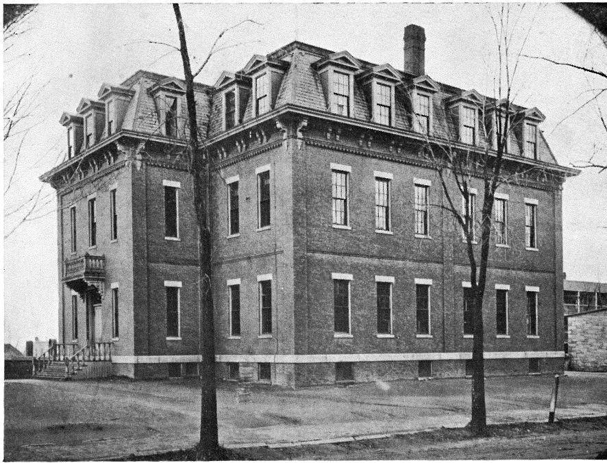
BATES STREET, COBURN SCHOOL
