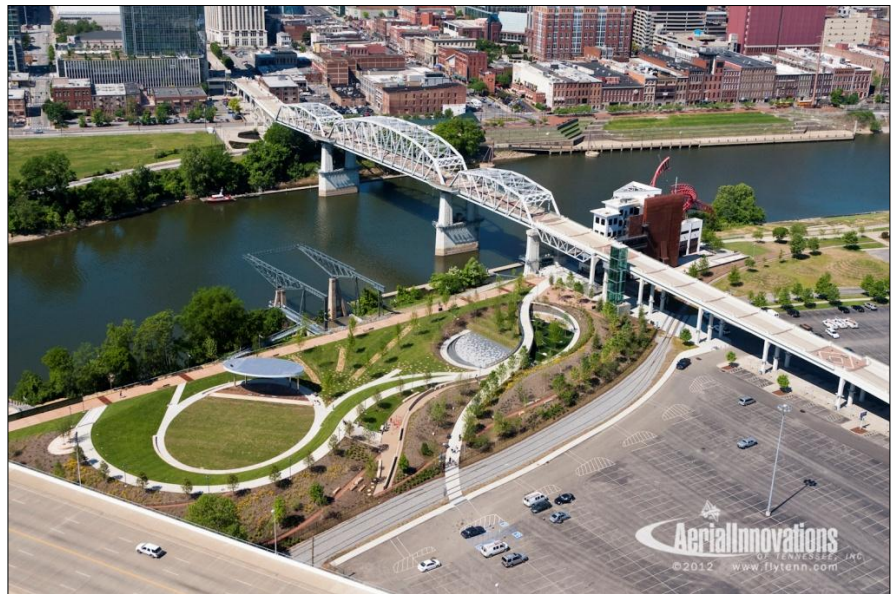
(above) A view of Cumberland park. Photo: Hargreaves Associates (below) Cumberland Park aerial view. Photo: Aerial Innovations.
