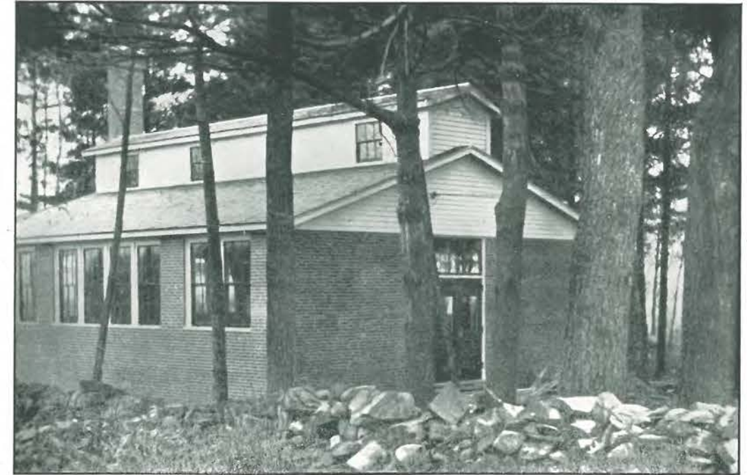
FORGE AND MACHINE SHOP
