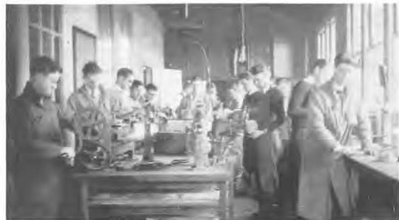
SHEET METAL SHOP
